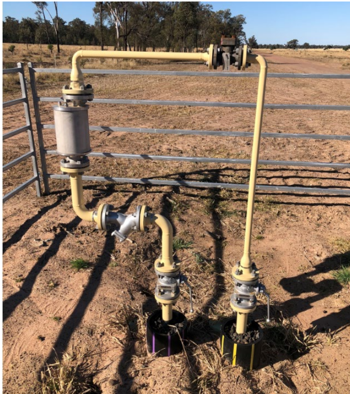
Plate 3-2 - Image of High Point Vent
