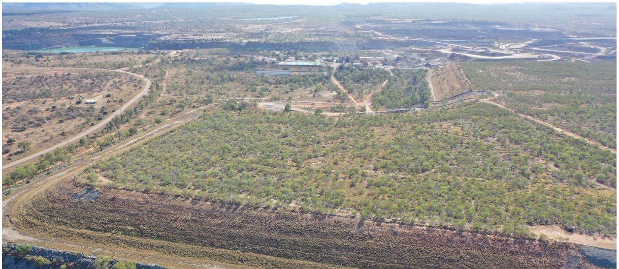
Figure 5. Established rehabilitation of the Tailings Storage Facility looking in a north-easterly direction towards the Sarsfield Pit.
