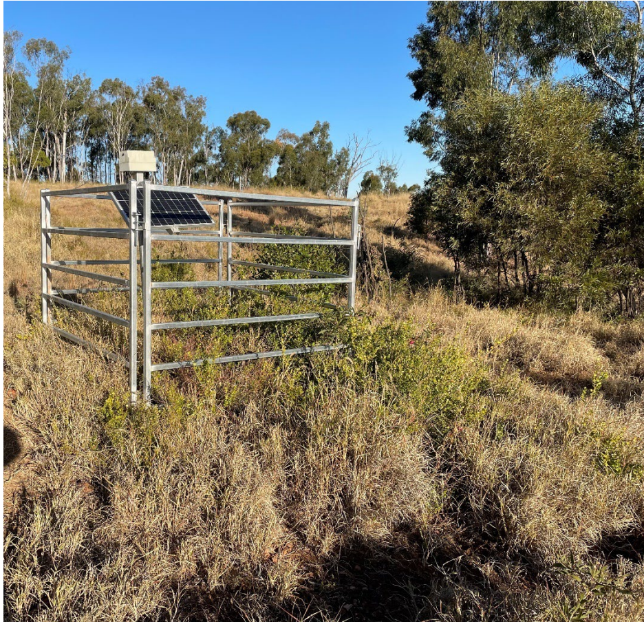
FIGURE 4-9 MONITORING STATION 114_1 PANEL.
