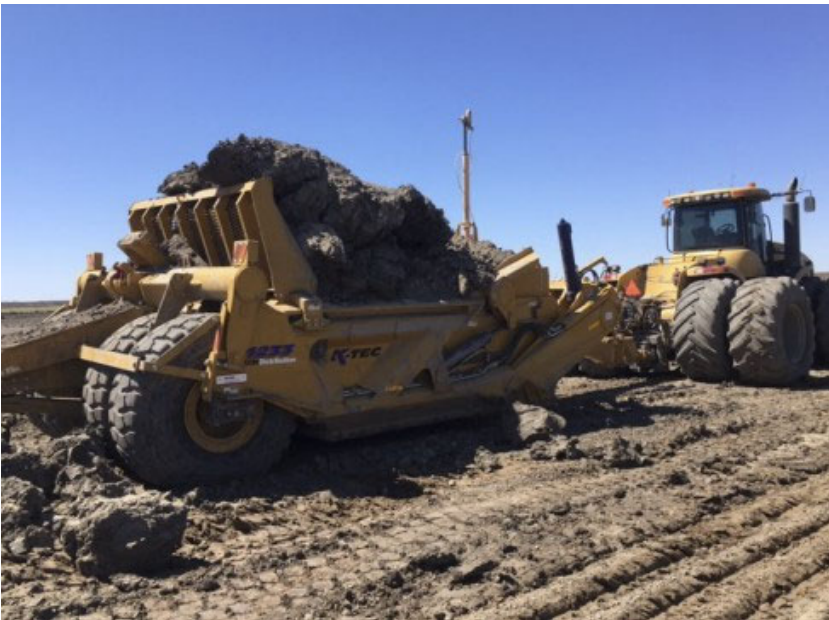
Figure 26 : Sub 2-3cm accuracies are unlikely to be achieved in situations like these due to cloddy or soft nature of soil (source: top – dryhireonline, bottom - Collier and Miller)
