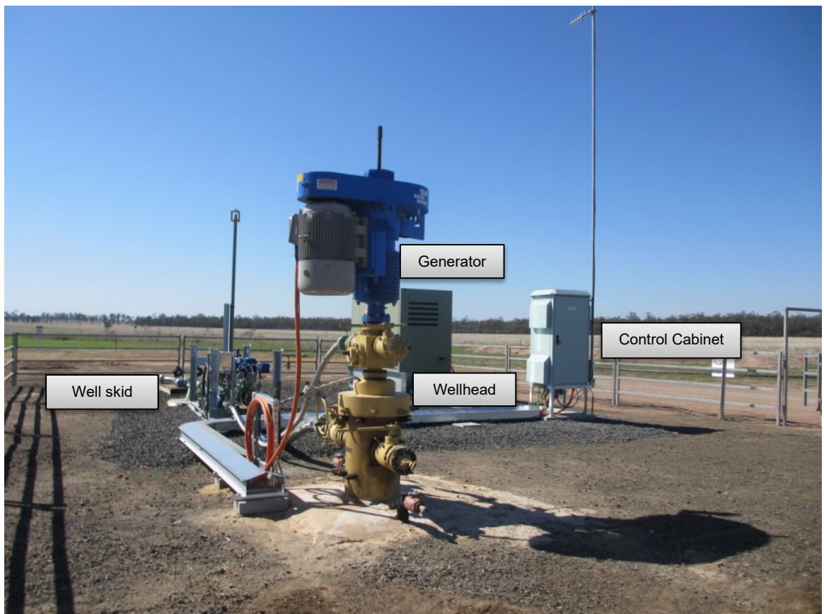
Plate 3-1 - Typical Well Head Facility and Infrastructure
