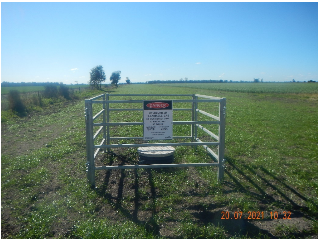
Plate 3-6 – Image of a valve and the ROW post reinstatement
