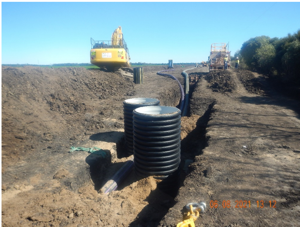
Plate 3-4 – Image of valves during construction within the ROW
