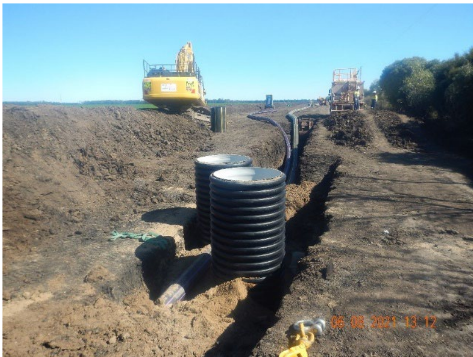
Plate 3-1 – Image of valves during construction
