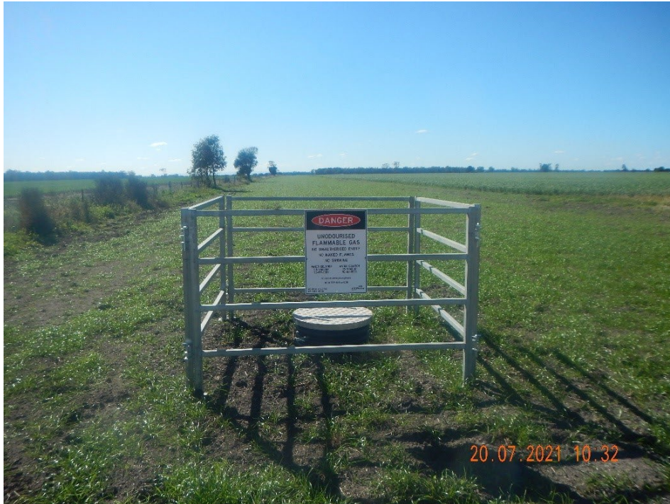
Plate 3-2 – Image of a valve post reinstatement
