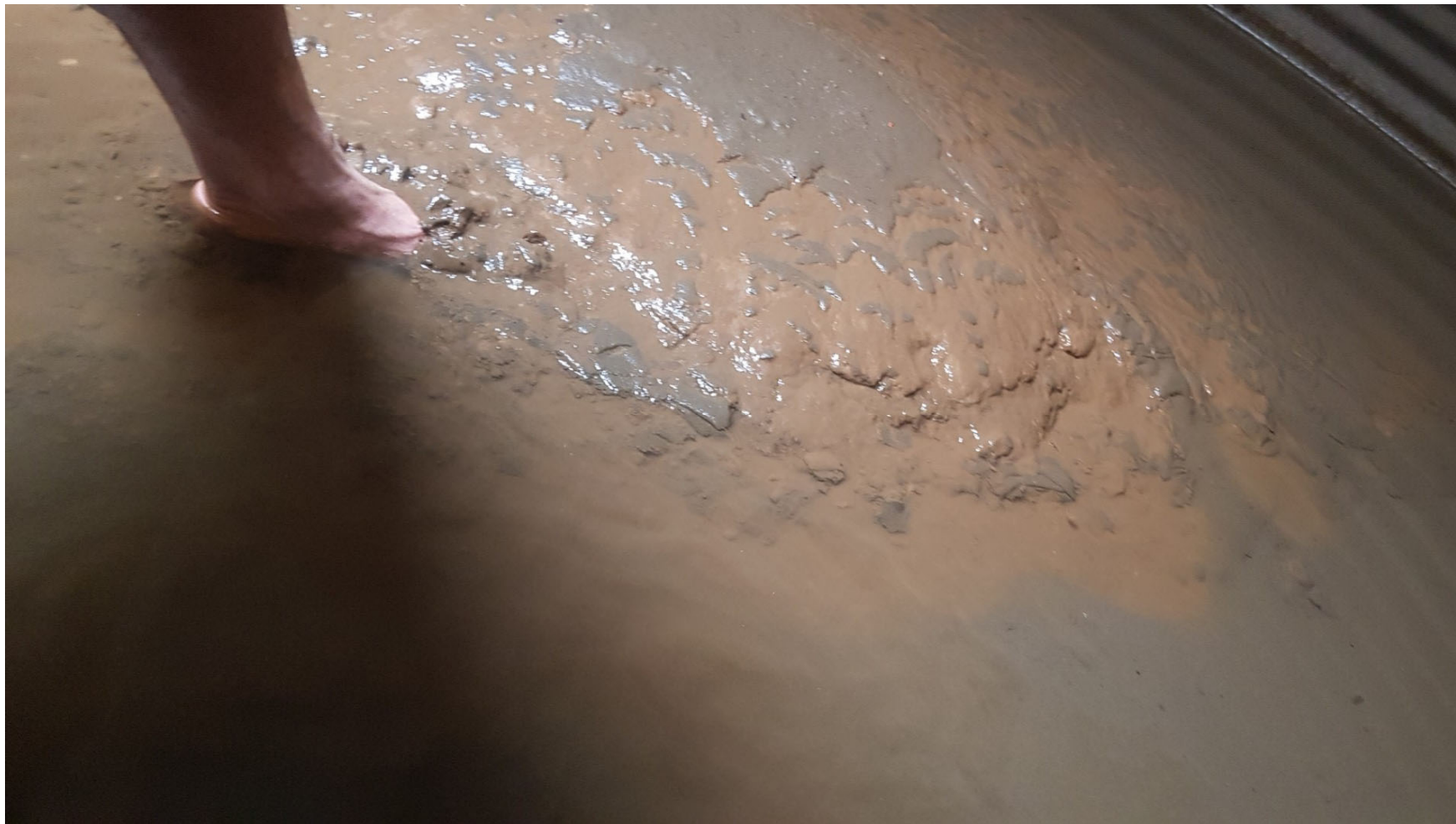
Figure – Water Tank [REDACTED] - Considerable Sludge Potentially from Resource Activities (Possible Dust & Blasting Fallout) – Cleaned 7/11/2022
